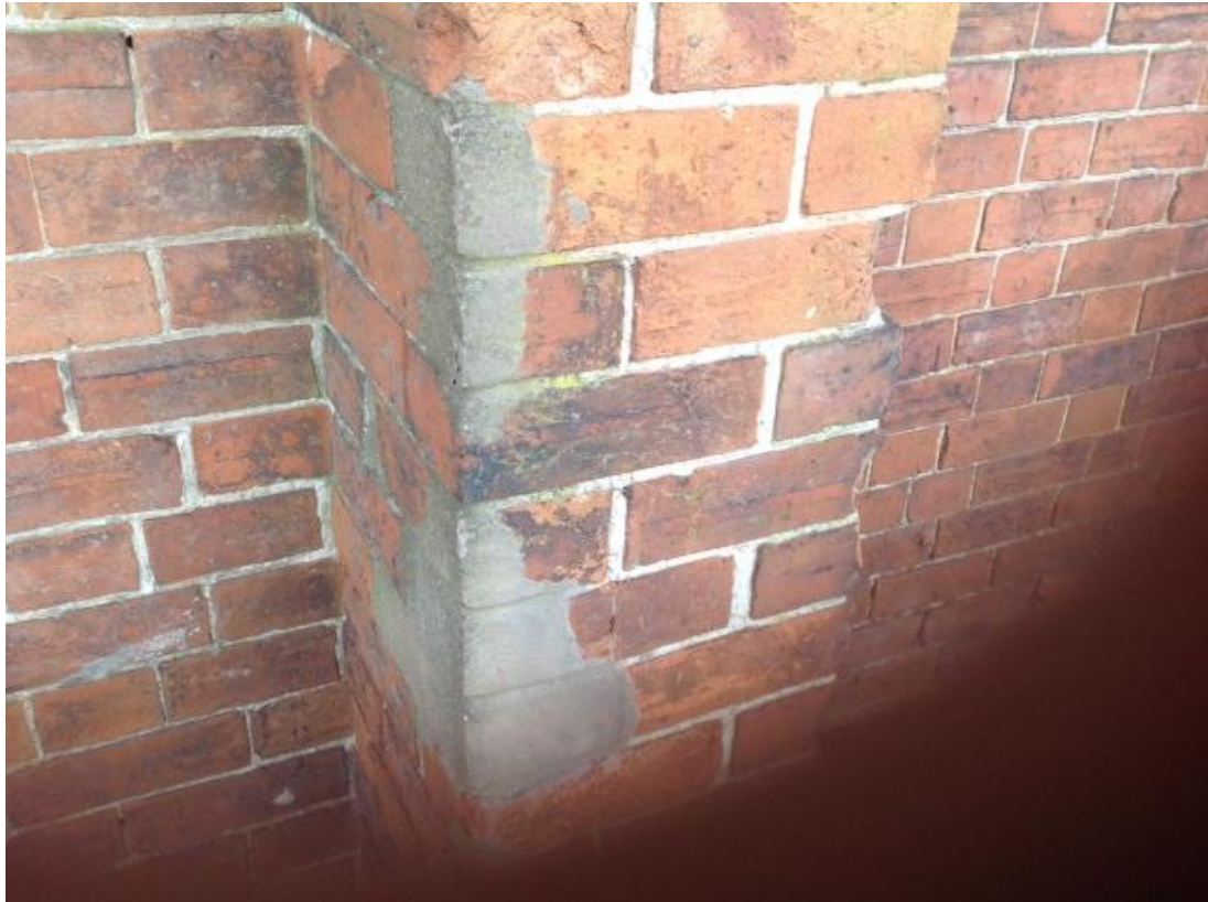
Image 12: Brick work pillar.
